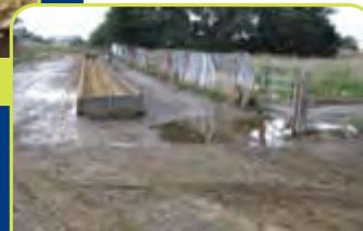
Concrete laneway with bins
