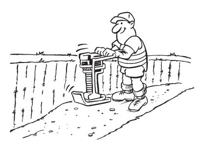
Compacted granular bedding/aggregate surrounds the pipe and up to a minimum 100mm above the pipe. Then I use selected ordinary backfill. I compact with my machine below, beside and above the pipe in layers of 300mm until I get to the top surface.
